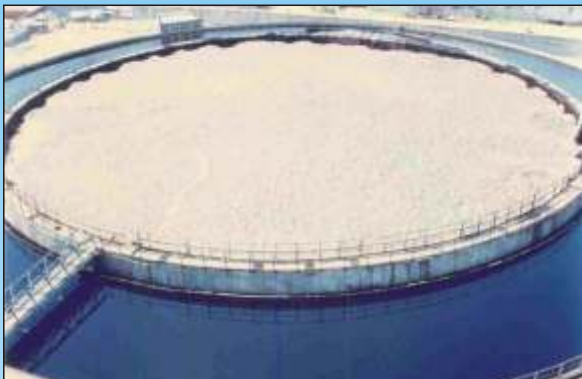
AERATION CUM CLARIFIER TANK AT CETP, VATVA - 16 MLD
