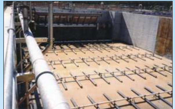
TYPICAL FIXED GRID DIFFUSED AERATION SYSTEM
